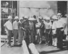
Trainees in the Utilities Training Program - Advanced I here listen attentively to Edgard Maduro of P. T. S. - Combustion Team, who is giving instructions on the use of oxygen analyzers. Here they are at Boiler No. 5 at Powerhouse # 1. Their training program was from March 20-April
